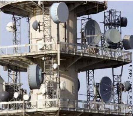
Telecom - Data infrastructure
